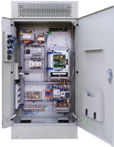
Close Loop (Integrated) Panel
